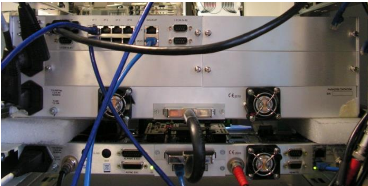
Figure 1-4 Redundancy Switch (showing connection to Backup Modem)
