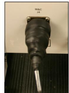
Prior to taping a connector, remove all traces of oil or grease from the connector by using an alcohol-based cleaning solution. Ensure the connector is clean and dry.
