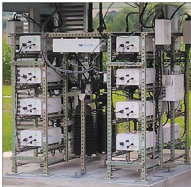
5 kW C-Band (16 Module) Outdoor PowerMAX System Using 400W GaN Compact Outdoor SSPA Package
