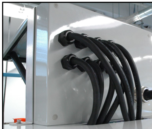
Figure 2-12: Insert Power Cables Through Top Cover Slot
