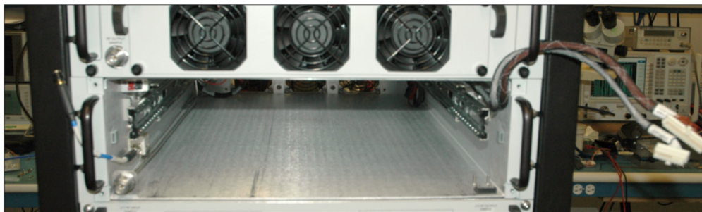
Figure 8: Shift Cables Out of the Way to Install Module/Heatsink Assembly
