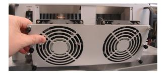
Figure 6: Remove Front Fan Assembly (5RU Chassis shown)
