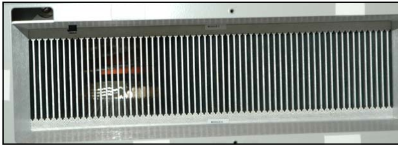
Figure 3-7: Heatsink Fins Cleared of Debris
